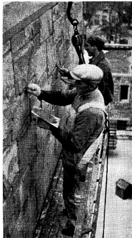
Pre-shrunk mortar placed properly in the joints
