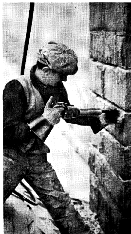
A Pneumatic Hammer Removes the bad Mortar
