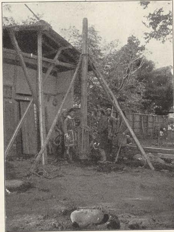
RAMMING THE GROUND FIRM
