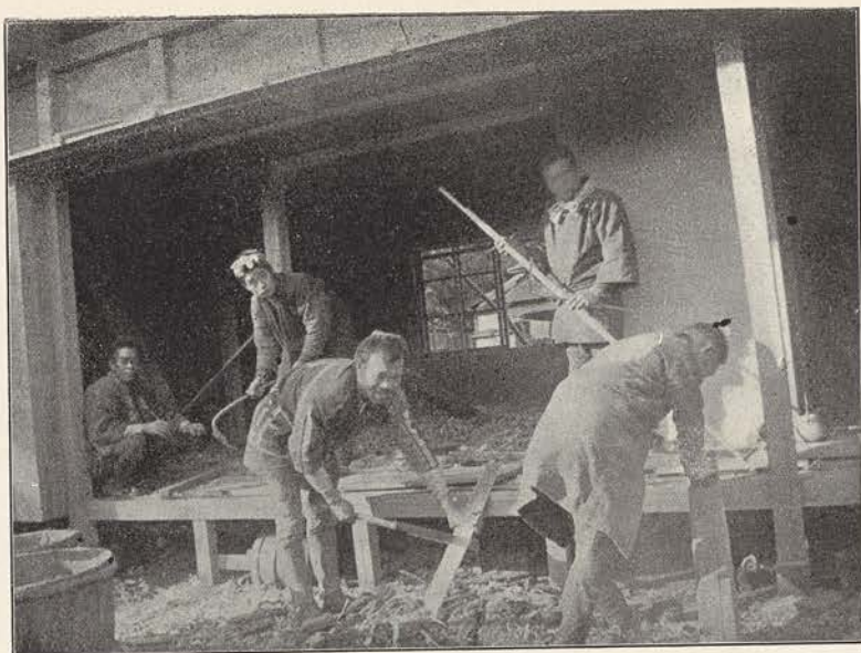
THE SENDAI CARPENTERS AT WORK
