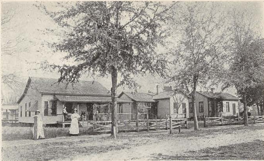
"FIVE SMALL ONE-STORY COTTAGES, UNFINISHED INSIDE AND OUT"
