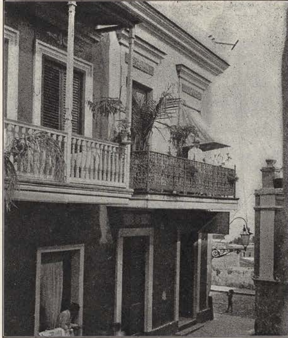
THE CORNER BUILDING IS THE BISHOP'S HIRED HOUSE, NO. 1, SANTO CRISTO STREET
