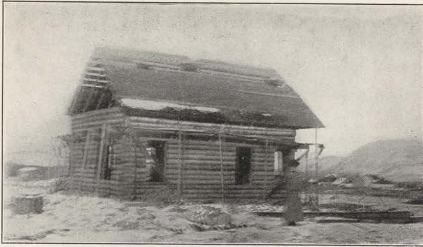
THE MISSION HOUSE NEARING COMPLETION
