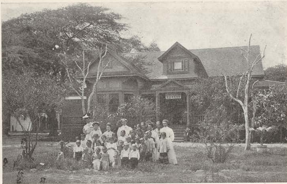
ST. MARY'S HOUSE
