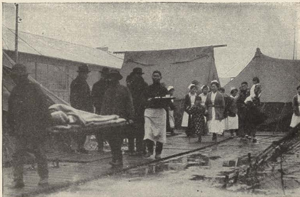
ST. LUKE'S HOSPITAL WORKS UNDER DIFFICULTIES
