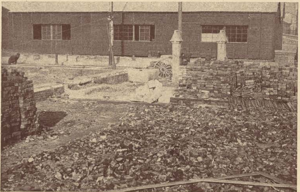
ALL THAT WAS LEFT OF ALL SAINTS' CHURCH The upright pillars alone are identifiable of what was among the most attractive of our churches in that city. The photograph shows how complete was the destruction
