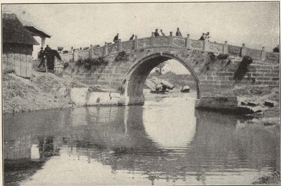
THE NORTH BOUNDARY BRIDGE BETWEEN SHASI AND KINGCHOW Here the Sisters of the Community of St. Anne change 'rickshas on the trip between the two cities. Simple but beautiful bridges like this are quite common in China
