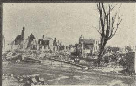
AFTER THE EARTHQUAKE - 1923
