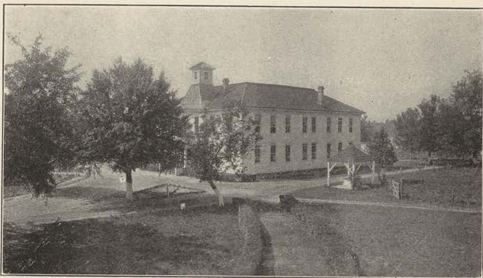
THE MAIN BUILDING OF VORHEES SCHOOL, DENMARK, SOUTH CAROLINA This is only one of the nineteen buildings large and small which represent the twenty-seven years of work done by the founders of this institution
