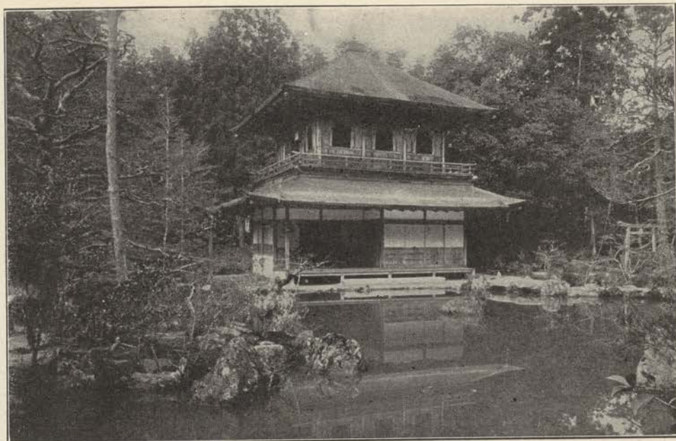
THE SILVER PAVILION, A PRINCELY PLEASURE HOUSE IN JAPAN The Province of Ise, in the district of Kyoto, abounds in such beautiful resorts for the wealthy. The building shown dates from 1479
