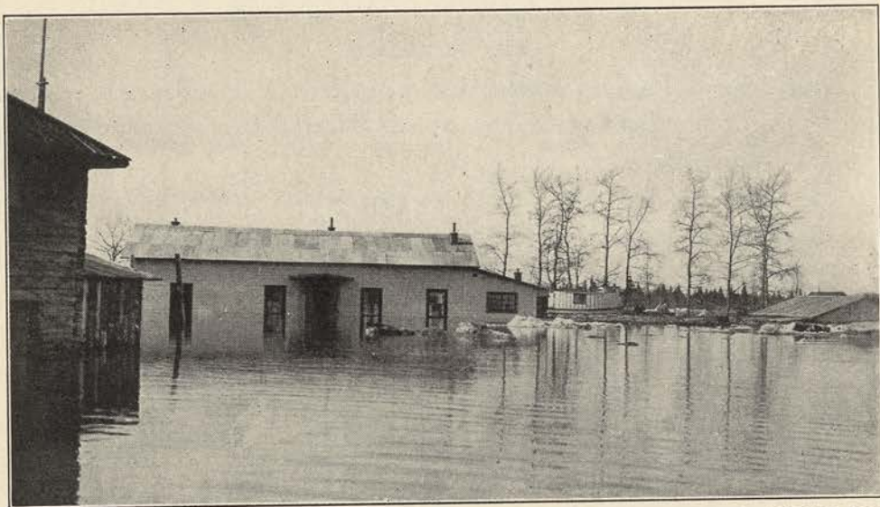
ONE OF THE BUILDINGS AT CHRIST CHURCH, ANVIK, SURROUNDED BY WATER
