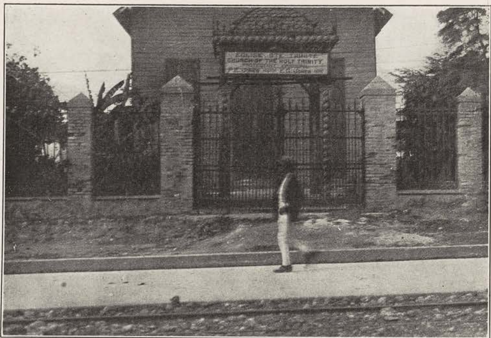
THE PRESENT CHURCH OF THE HOLY TRINITY, PORT AU PRINCE Never a substantial building, this Pro-Cathedral of our Church in Haiti is almost ready to fall to pieces. $12,500 of the Corporate Gift will help build a new church
