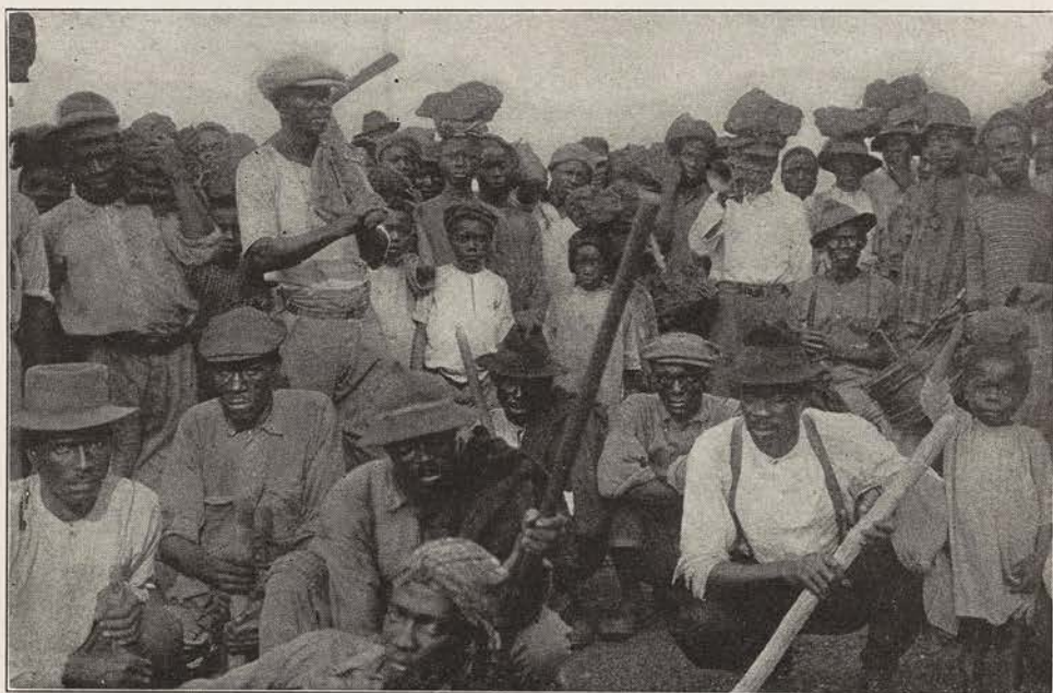
VOLUNTEERS AT WORK ON THE CAPE MOUNT HOSPITAL
