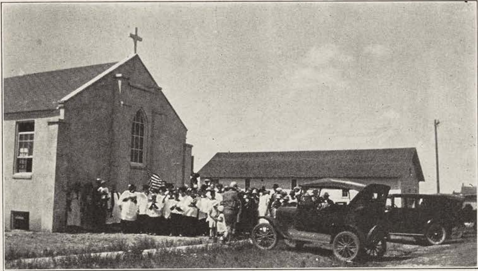
AFTER THE OPENING SERVICE IN THE NEW CHURCH AT DUPREE The first services were held in Dupree a very few years ago and the mission has had many discouragements, but it has succeeded in building this beautiful little church
