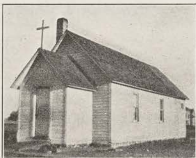
GUILD HALL AT DUPREE Transformed into a comfortable rectory when the new Church was built
