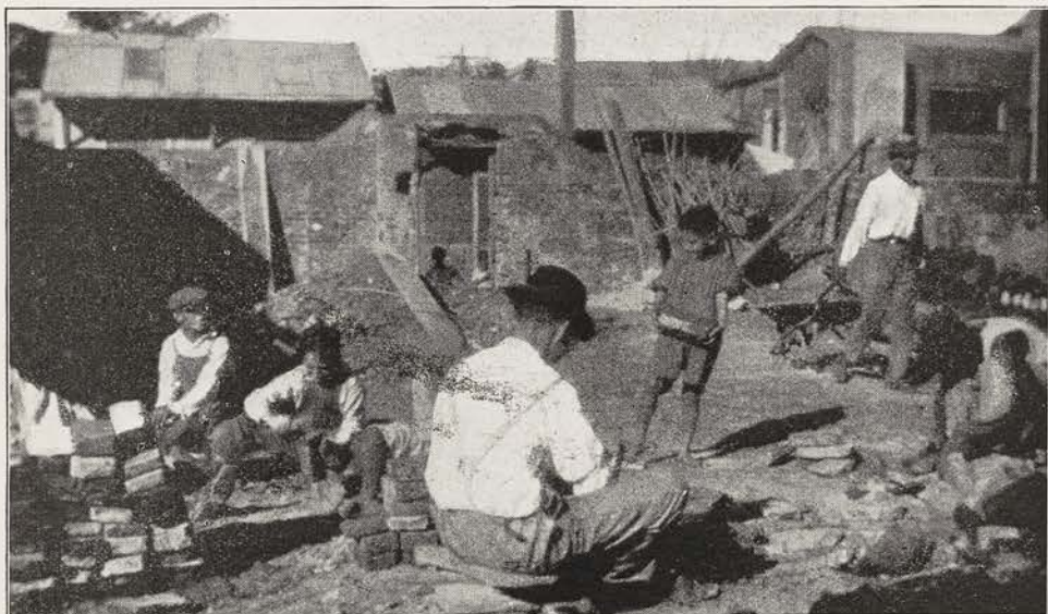
SEÑOR VILLAFANE AND HIS BOYS GETTING THE GROUND READY FOR THE PLAYGROUND AT ST. ANDREW'S SCHOOL, MAYAGUEZ, PORTO RICO
