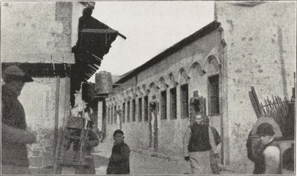
ST. ANDREW'S CHURCH IN A SUBURB OF WUCHANG WHERE A MACHINE GUN, OPERATED FROM THE NAVE, WAS STATIONED ON THE PORCH
