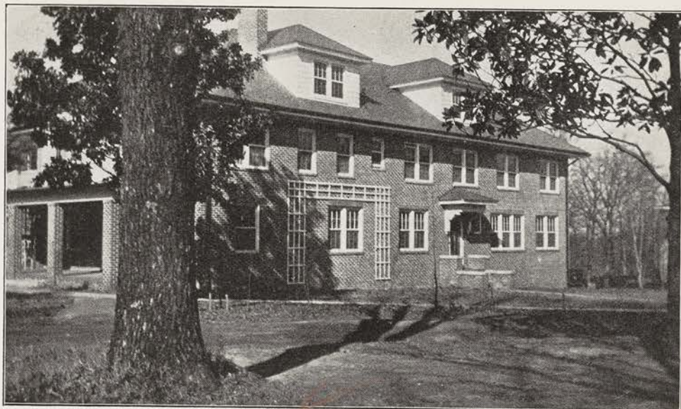
THE BISHOP TUTTLE MEMORIAL HOUSE FOR TRAINING COLORED CHURCHWOMEN Located on the campus of St. Augustine's School, Raleigh, N. C., on ground donated by the Rev. Dr. Hunter and Mrs. Hunter, this house fills a need which has been long felt
