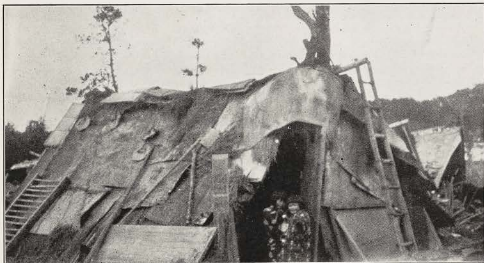
TEMPORARY HOME OF EARTHQUAKE SUFFERERS IN THE TANGO DISTRICT
