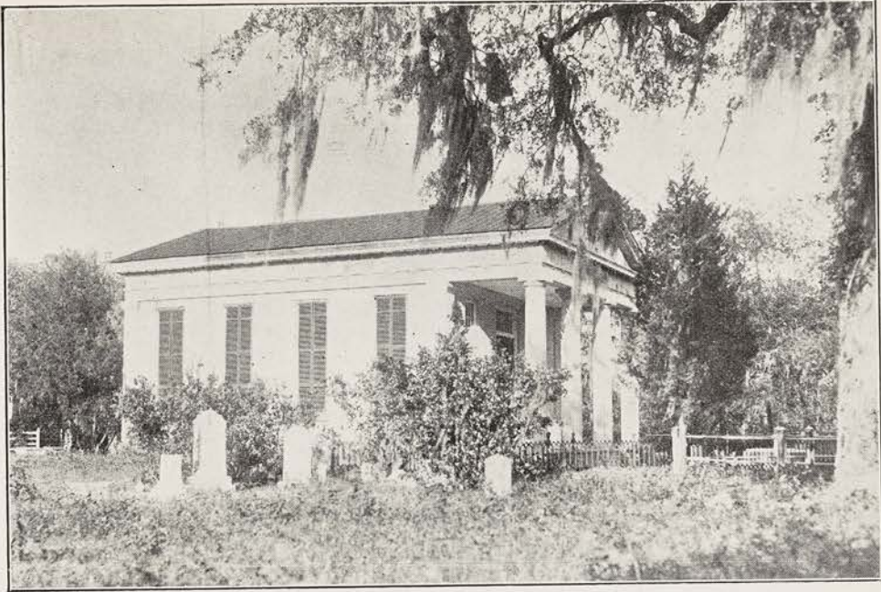
CHURCH OF PRINCE GEORGE, WINYAH, PARISH, GEORGETOWN, SOUTH CAROLINA This parish was founded in 1721 by the Colonial Council of South Carolina, which appropriated a thousand pounds for a church. This building was completed about 1750
