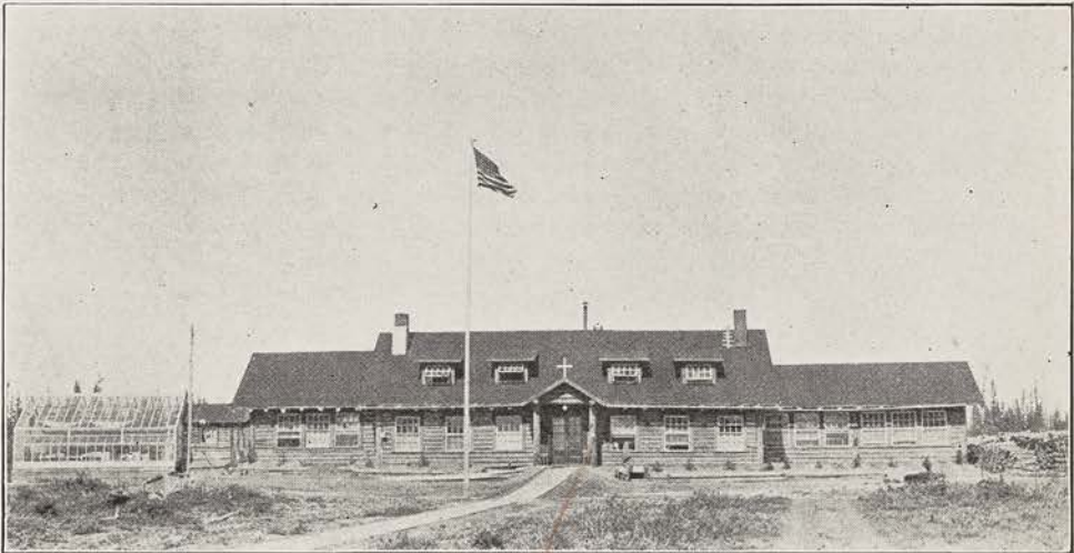
THE HUDSON STUCK MEMORIAL HOSPITAL, FORT YUKON, ALASKA
