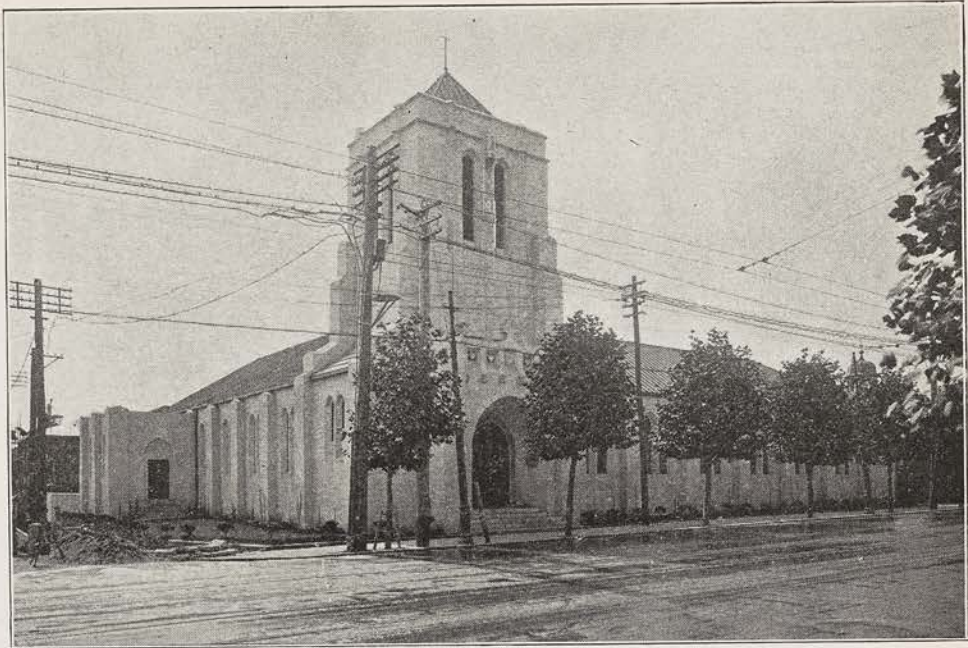
THE NEW HOLY TRINITY CATHEDRAL, TOKYO, CONSECRATED OCTOBER 17, 1927 Replaces the church destroyed in the great earthquake of 1923. It is entirely built of reinforced concrete to withstand future earthquakes, and is directly opposite one of the Imperial palaces
