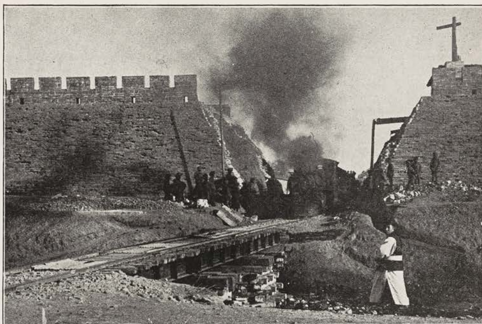
A NEW CIVILIZATION IS BREAKING DOWN ANCIENT BARRIERS IN CHINA The wall surrounding the City of Peking, built in 1543, is twenty-five feet thick at the base and thirty feet high. A breach was made in it to allow the railroad to pass through.
