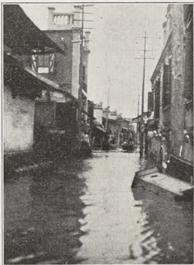
FLOODED STREET IN CH'UCHOW The water is ten feet deep. Note the police sentry box floating away
