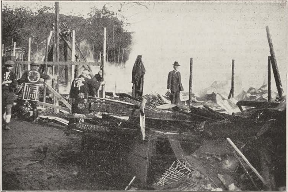
RUINS OF THE LABORERS' REFORM UNION WORKSHOP, TOKYO Mr. Sugiura is seen in the center of the debris. He said, "There was a moment when I was at a loss as to what to do, but God helped me"
