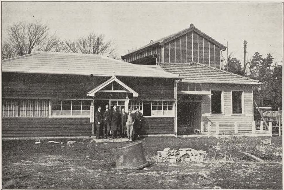
NEW WORKSHOP OF THE LABORERS' REFORM UNION, TOKYO The new building at Higashi Nakano which is partly completed and where part of the work is already being carried on, thanks to friends who came to the rescue
