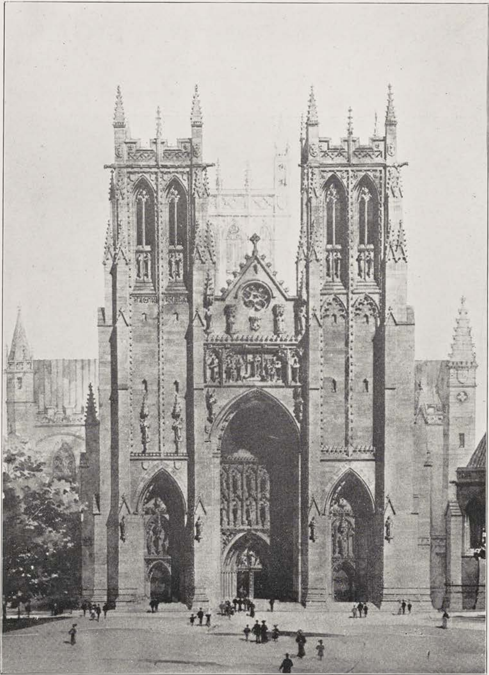
FACADE OF WASHINGTON CATHEDRAL FROM ARCHITECT'S DRAWING Showing the two western towers as they will appear when completed. The great central tower, seen in the background, is 262 feet high. The western towers will rise to 196 feet
