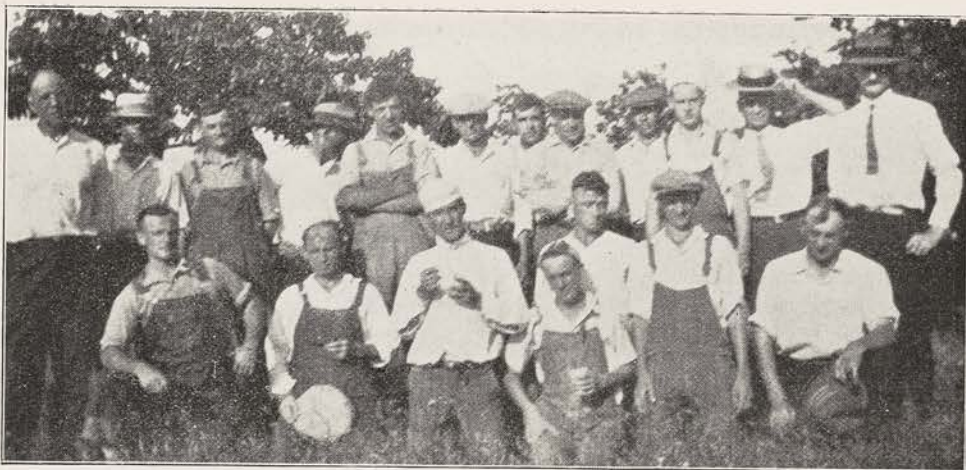
THE MEN OF ST. MARK'S MISSION, WEST FRANKFORT, ILLINOIS Wanting to help but having very little to give, the men of the congregation put the shingles on the church on days when the mines were not working
