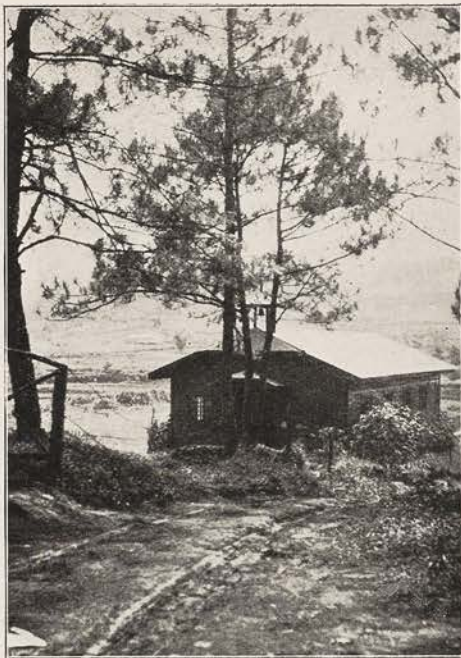
TEMPORARY CHURCH OF THE RESUR- RECTION, BAGUIO
