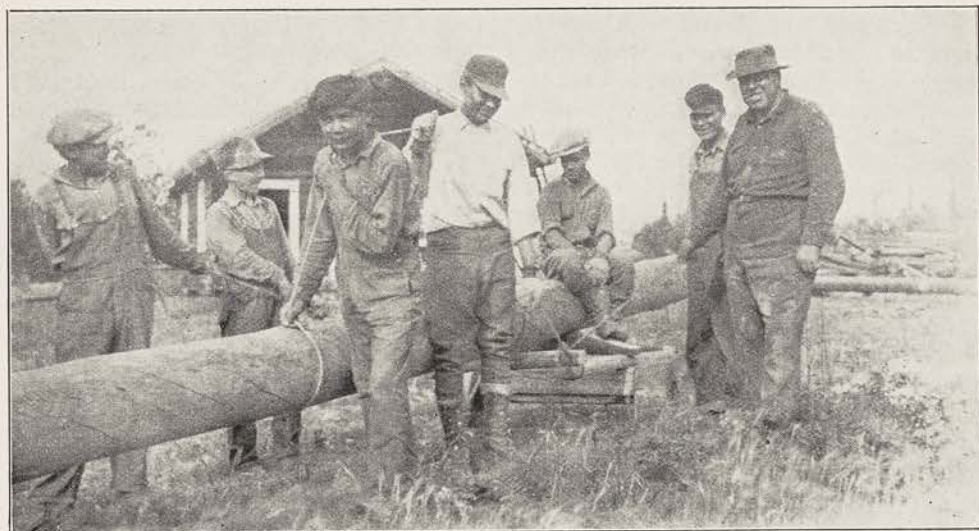
MOVING THE MISSION HOUSE AT STEPHEN'S VILLAGE TO TANANA Mr. Nicholson, the contractor who has been so helpful to our Alaska missions, stands at right. The house was taken down and the logs rafted down the Yukon.
