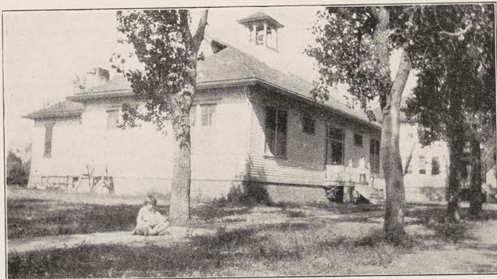
CROW CREEK DORMITORY, FORT THOMPSON, SOUTH DAKOTA
