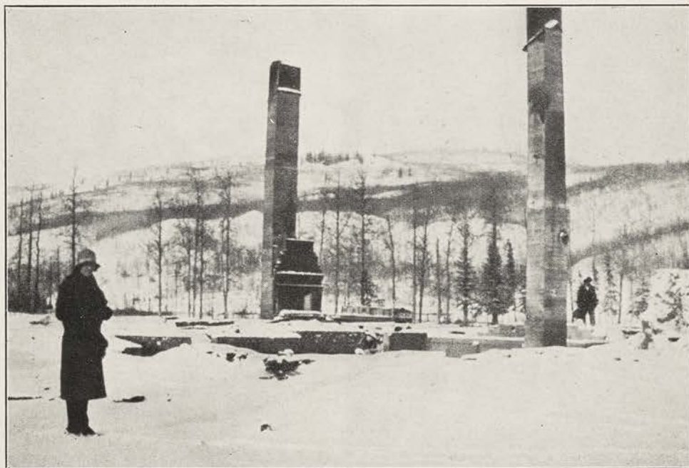
AFTER THE NENANA FIRE OF JANUARY 23 In addition to the complete destruction of the building, some equipment together with the personal belongings of the mission staff and school children, were lost
