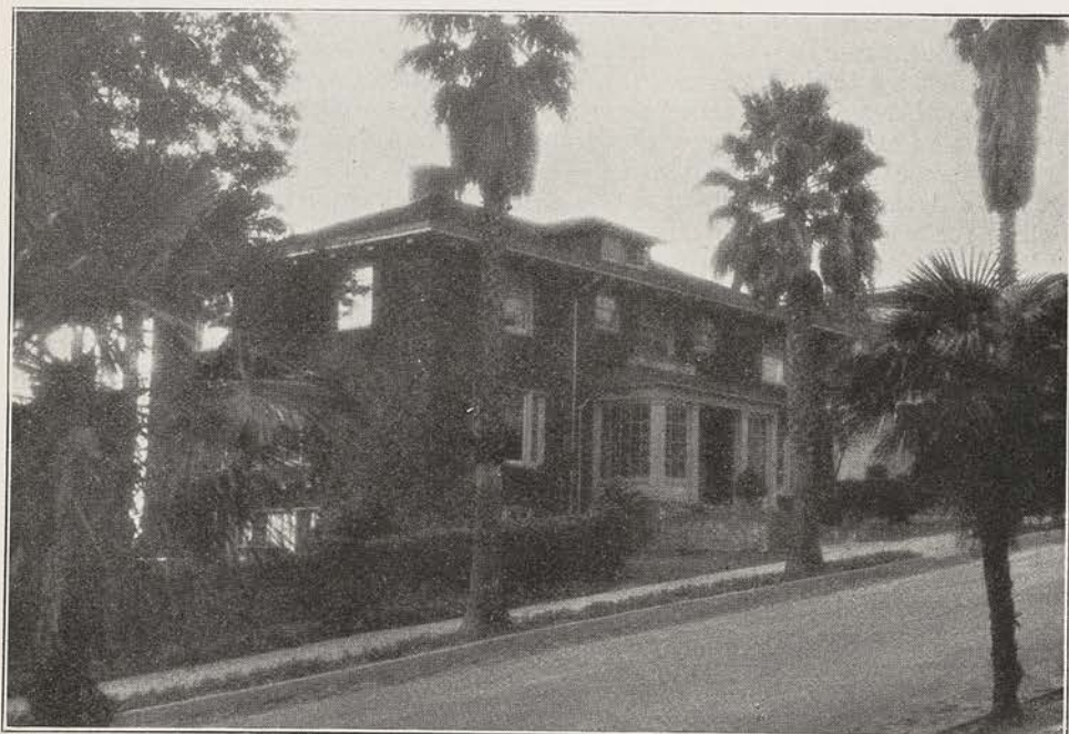
THE NEW ST. MARGARET'S HOUSE, BERKELEY, CALIFORNIA Made possible by a grant from the United Thank Offering and additional gifts, the new house is strategically located in relation to the Pacific School of Religion and the University of California. A wing providing dormitory accommodations is under construction
