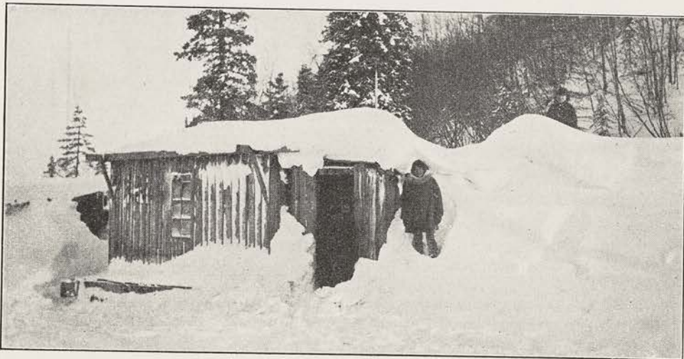
THE CHURCH'S FIRST HOUSE IN ANVIK
