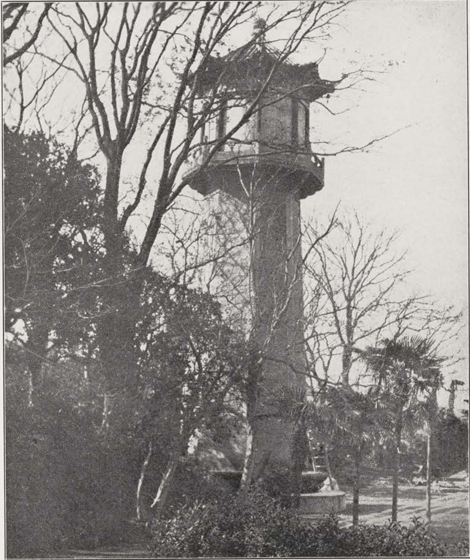
WATER TOWER, HUA CHUNG COLLEGE, WUCHANG
