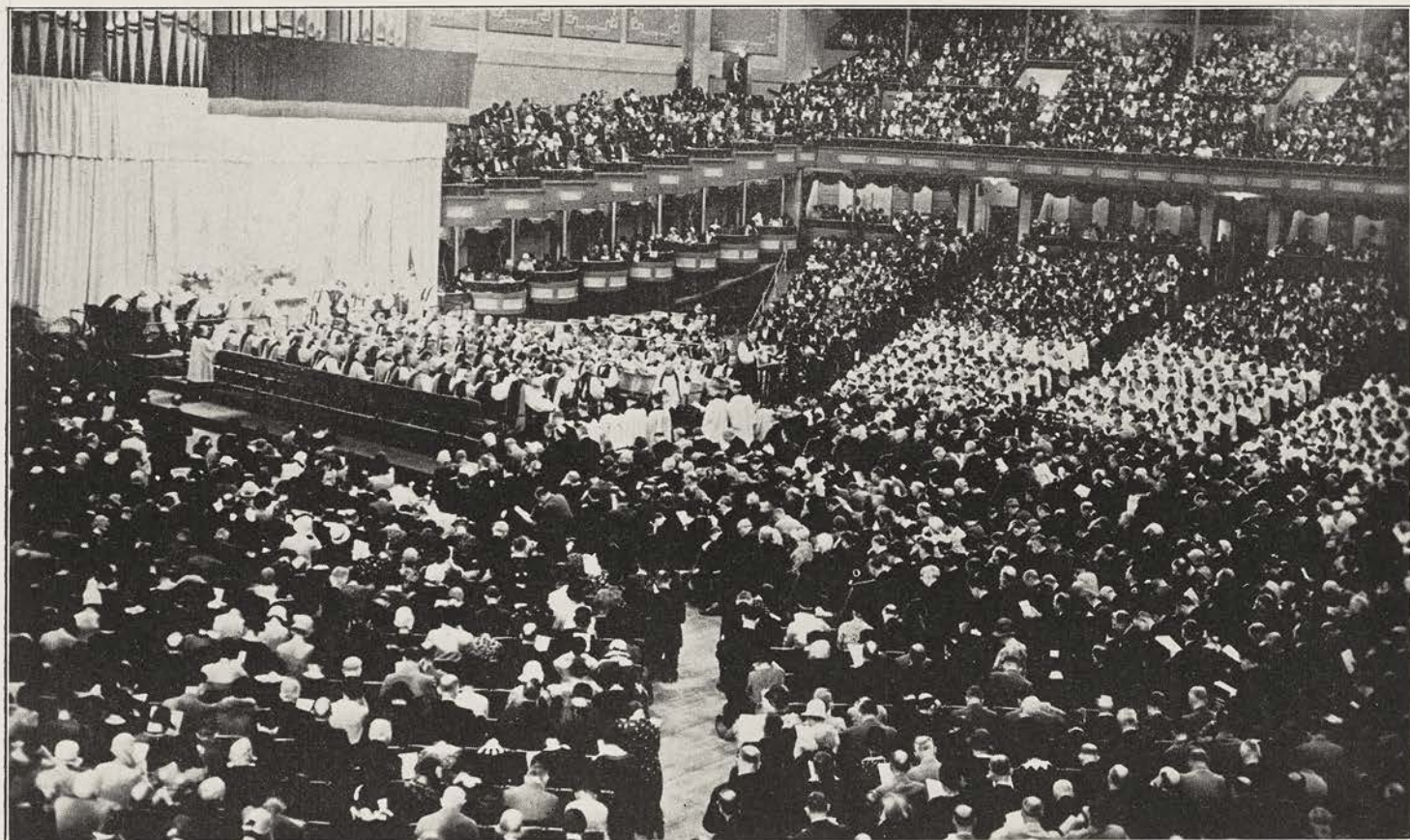
OPENING SERVICE, FIFTIETH GENERAL CONVENTION, MUNICIPAL AUDITORIUM, DENVER, COLORADO, SEPTEMBER 16, 1931 Distinguished Churchmen from all over Christendom filled this huge auditorium for the opening of a memorable Convention
