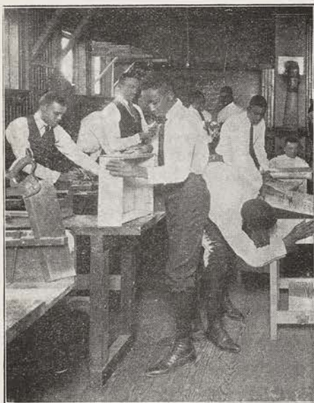
ELEMENTARY CABINET MAKING Future craftsmen receive vocational training in St. Paul's, Lawrenceville
