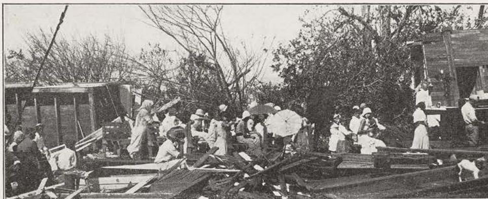
LA GLORIA CONGREGATION GATHERS FOR SERVICE AMID THE RUINS OF THEIR CHURCH
