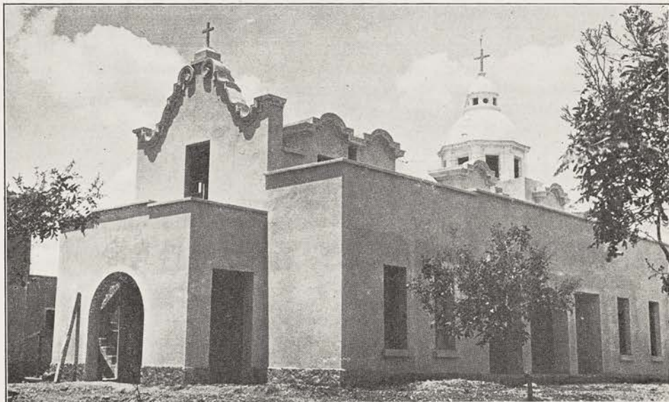
THE NEW CHAPEL FOR ST. ANDREW'S SCHOOL, GUADALAJARA, NEARS COMPLETION Bishop Salinas y Velasco was in charge of this school prior to his elevation to the episcopate. The school which is now in charge of the Rev. L. J. Saucedo has about twenty pupils
