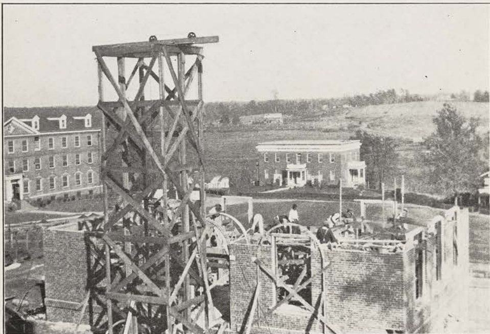
NEW ADMINISTRATION BUILDING RISES AT ST. PAUL'S SCHOOL, LAWRENCEVILLE
