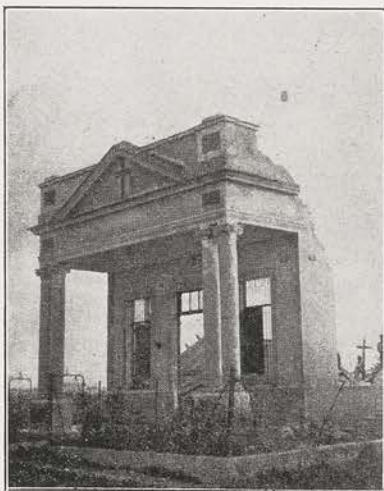
AFTER THE HURRICANE: THE REMAINS OF GOOD SHEPHERD CHURCH, WOODIN
