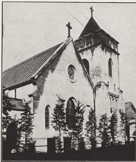
CHRIST CHURCH, KANDA, TOKYO Erected with the help of the Church in America, this fine plant replaces one destroyed by the 1923 earthquake
