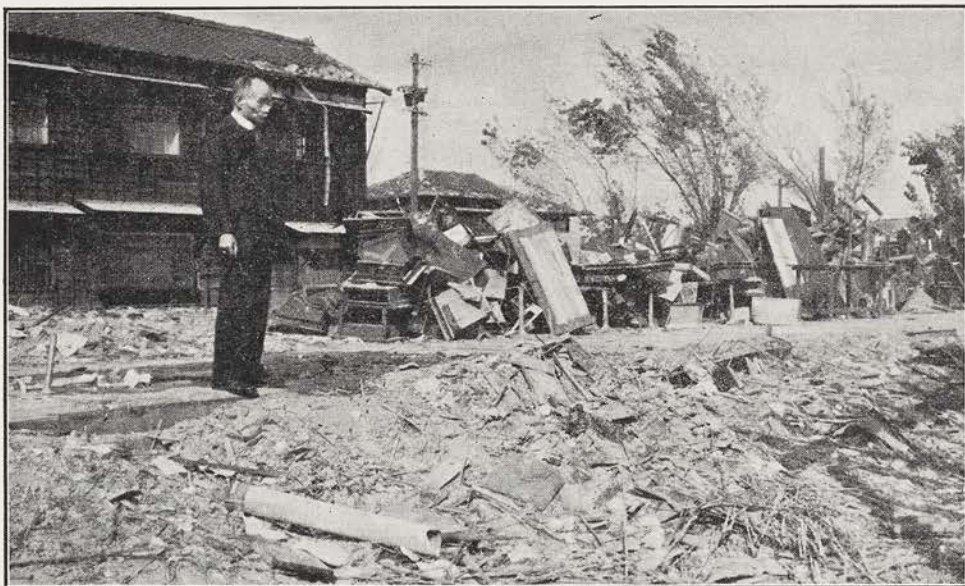
BISHOP NAIDE AT SITE WHERE POOLE SCHOOL CLASSROOM COLLAPSED Seventeen girls were killed and thirty-two injured when the September typhoon wrecked a part of this Osaka Church institution
