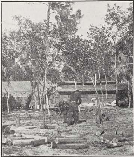
TRANSIENT WORK PROJECT
