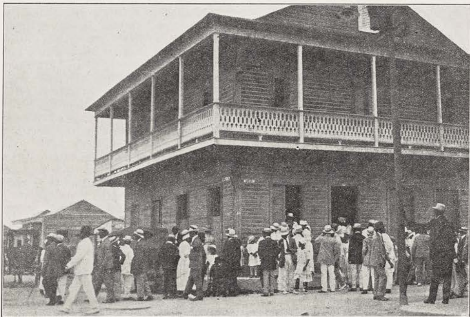
ST. STEPHEN'S MISSION, SAN PEDRO DE MACORIS, DOMINICAN REPUBLIC The dilapidated frame building which is the center of the Church work in Santo Domingo. The first floor is used for a church and the second as the home of the missionary, the Rev. A. H. Beer (see page 513)
