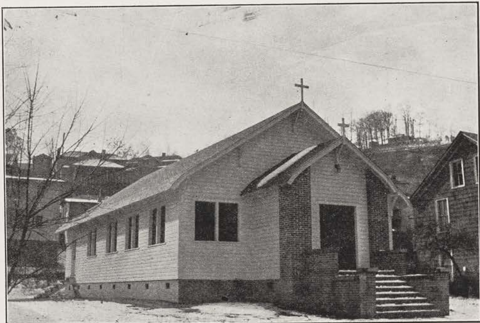
THE NEW CHRIST CHURCH IN PIKEVILLE, KENTUCKY This building made possible through a gift from the Woman's Auxiliary of the Diocese of New York, replaces a grocery store as a place of worship for the mountain congregation which is in charge of the Ven. Gerald H. Catlin
