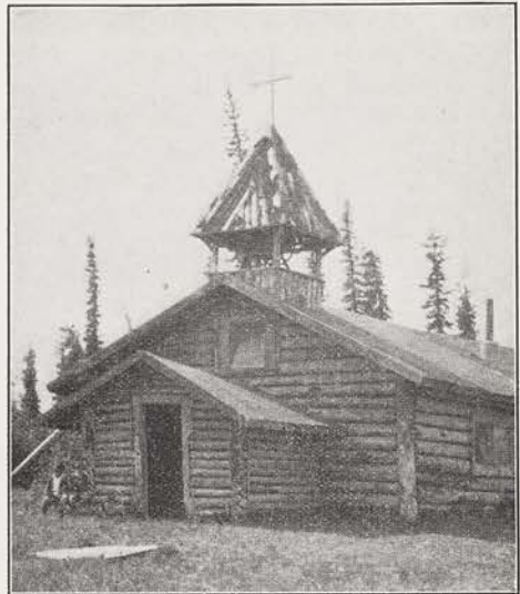
ST. JOHN'S, ALLAKAKET
