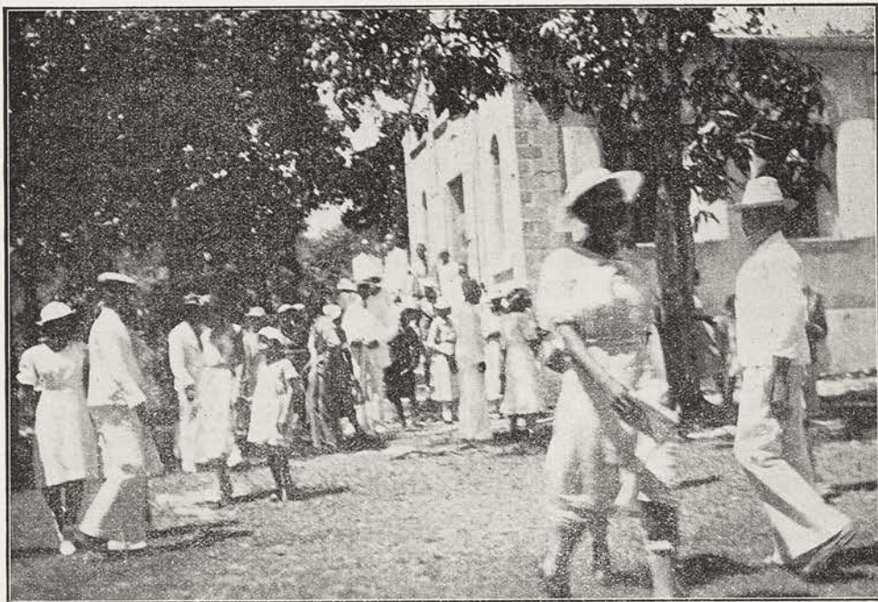
SERVICE IS OVER, ASCENSION CHURCH, THOR, HAITI
