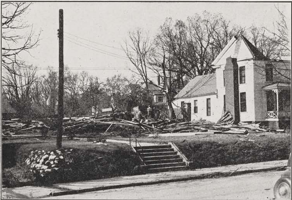
GRACE CHURCH, GAINESVILLE, GEORGIA, DEMOLISHED BY TORNADO During the storms which recently visited the Southern States, this century-old church was leveled to the ground and the rectory next door was badly damaged. The congregation numbers forty-six communicants
