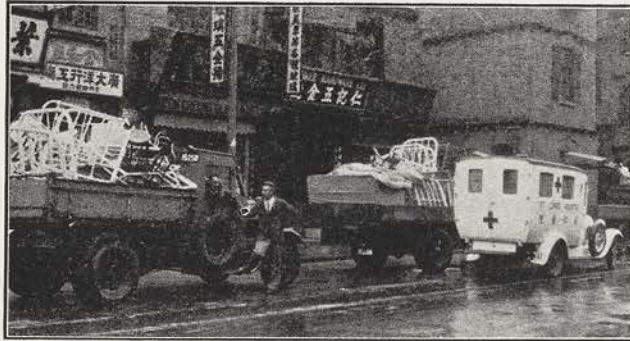
St. Luke's Hospital moves from Hongkew to safer quarters
