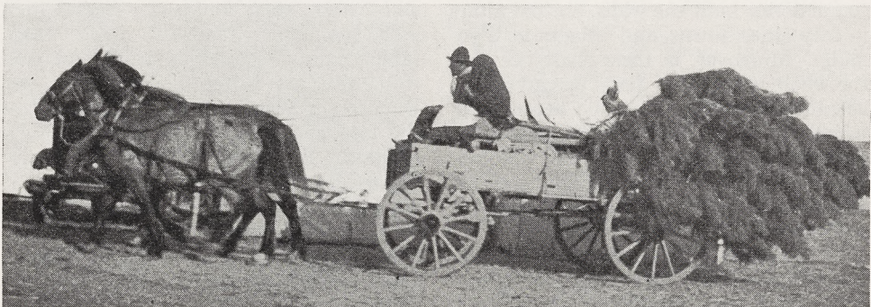
HOMEWARD BOUND , Convocation over, tents came down, trucks and wagons were loaded and the homeward way begun. This family is taking home some of the branches used on the Booth
